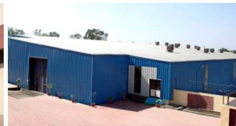
BOOSTER & OPENWELL / MONOBLOCK PLANT
